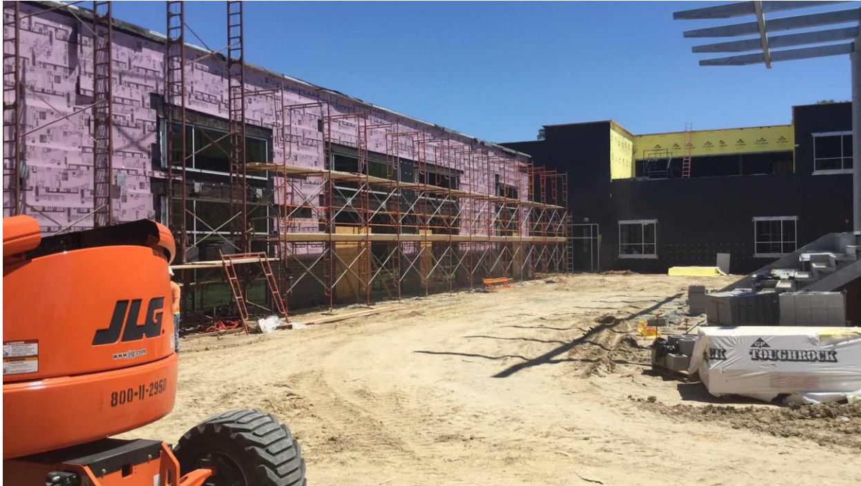
Building C – Rigid Insulation & Brick
