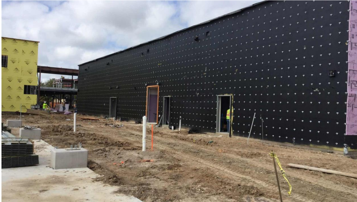
Building C – Waterproofing & Brick Ties
