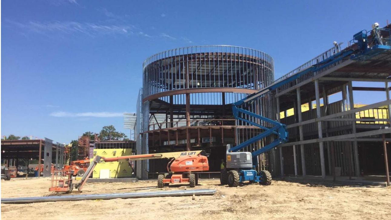
Building B – Radius Studs
