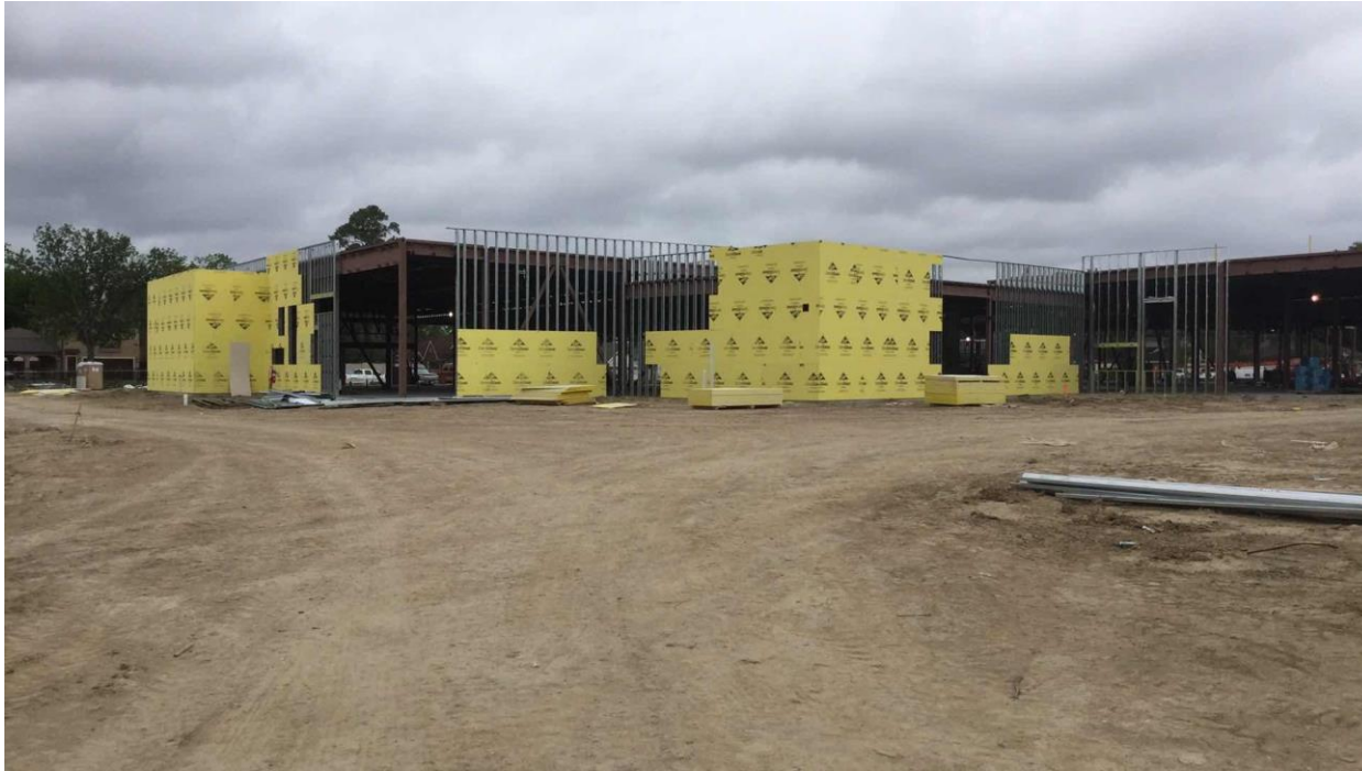
Building A – Sheathing & Studs
