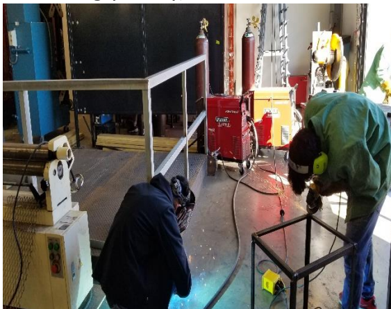
Welding (FCAW), Oxygen Fuel Cutting (O
